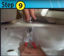
Secure the seat using pliers... DO NOT OVER TIGHTEN. \*Left / Right Hinges - Refers to the left and right mounting holes on the toilet when facing it.
