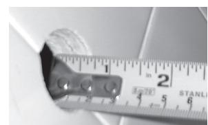
8. Measure the thickness of the wall by inserting a tape measure into the 1-1/4" (30mm) hole.
