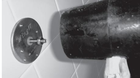
14. Verify the length of the nut from the **WingIt™** faceplate is correct (step 8) – Then hit the **WingIt™** firmly with a rubber hammer.
