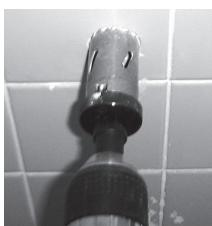
3. Carefully drill a 1-1/4" (30mm) hole in the wall precisely at the center point where each grab bar flange will align. In Ceramic Tile a piece of masking tape over the tile helps the drill bite into the tile. For Ceramic Tile an Industrial Grade Carbide Tip Hole should be used.
