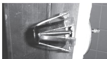
Picture Above Shows the inside of the wall after the **WingIt™** has been installed.
