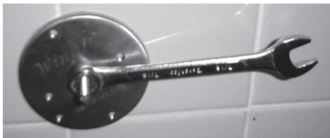
15. Pull on the bolt and tighten the nut by hand.
