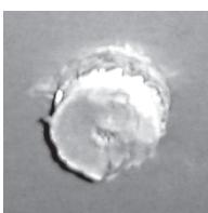
6. Then carefully finish the 1-1/4" (30mm) hole through the drywall. Do not push the drill. Allow it to cut, keeping the drywall intact behind the wall.
