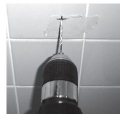
2. Use a 1/8" (3mm) drill or punch to make a starter/pilot hole. Once the first pilot hole is drilled check your measurement to the other hole.
